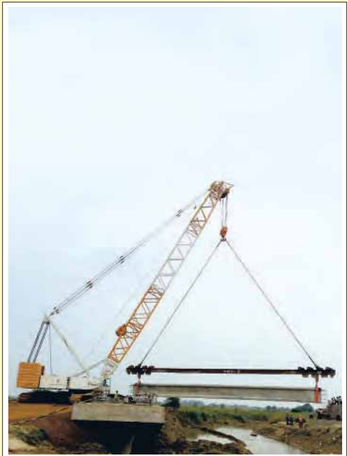
DEMAG CC 2400 (Capacity 450 MT) Crawler Crane, main boom 36M erecting Bridge Girder 80 MT at Afcons Infrastructure Limited site at Etawah, Uttar Pradesh
