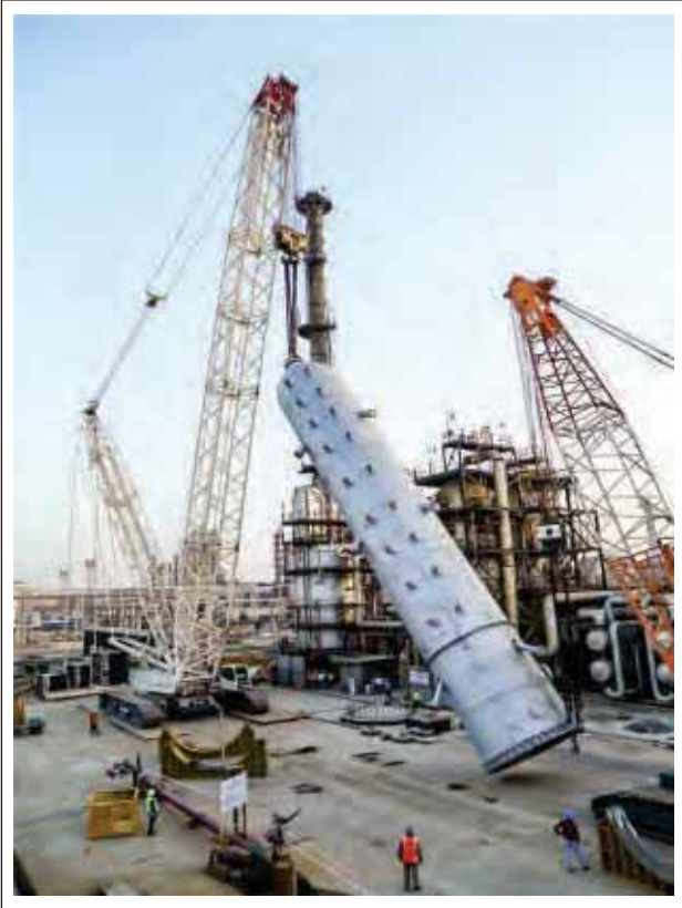
TERREX DEMAG CC 2400-1 (Capacity 400MT) Crawler mounted lattice boom Crane in SSL- 48Mtrs configuration erecting column of 210MT at KKSEPL, IOCL VADODRA
