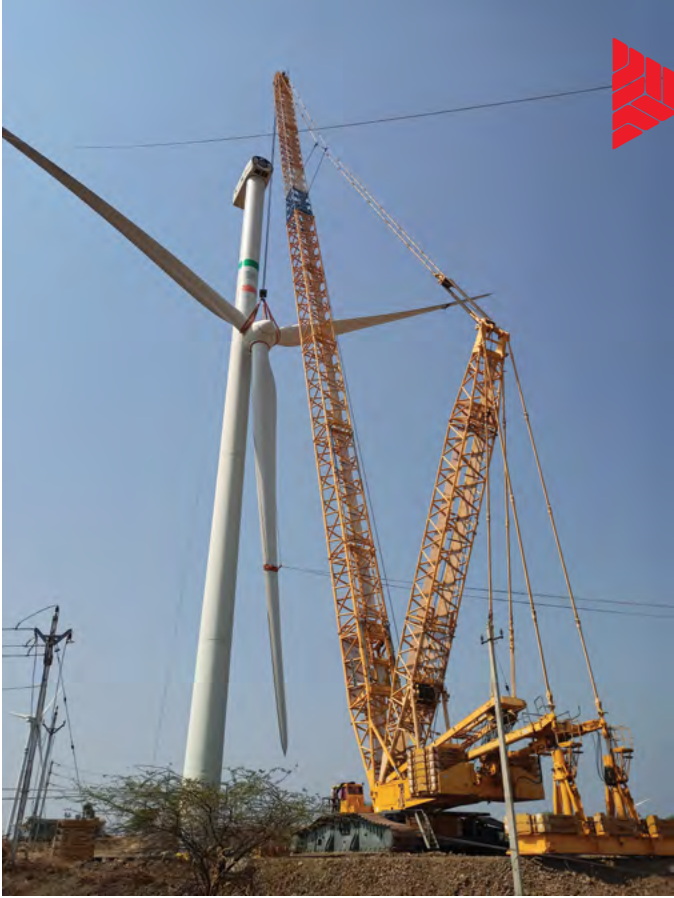
LR1750 (750 MT Crane) lifting Windmill rotor at Bangewadi, Karnataka
