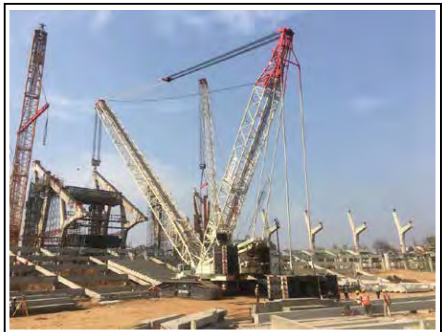
Terex -Demag CC 2800-1 working in Motera Cricket Stadium at Ahmedabad, GJ.
