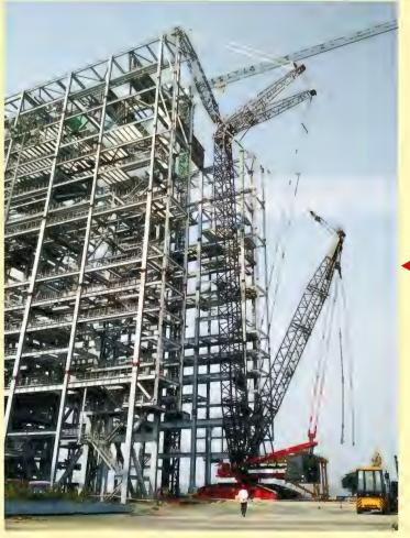
LIEBHERR LR1800 (Capacity 800MT) Crawler Crane, Erection of CEILING GIRDER of Weight – 212MT at Height – 90m with Crane Configuration SDW 70m + 42m for 2 x 660MW Lanco Vidarbha Thermal Power Project, Wardha, Maharashtra.
