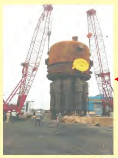
MANITOWOC M250S2 (Capacity 275MT) Crawler Crane, Tandem Lifting of REGENERATOR HEAD for CYCLONE Assembly of Weight 280MT with TWO nos of MANITOWOC M250S2 cranes at L & T Heavy Engineering, Hazira, Gujarat.
