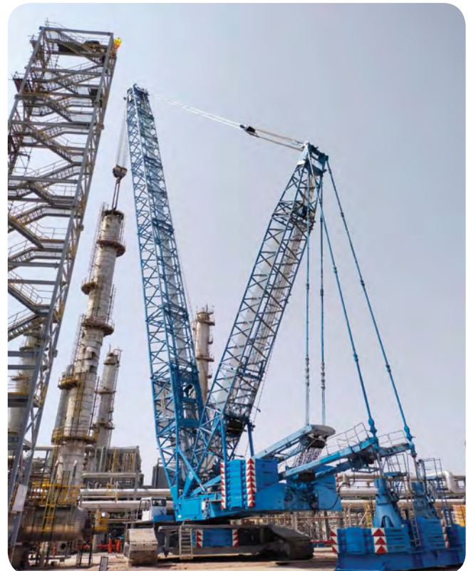
Liebherr LR 1750 – 750 MT successfully completed shutdown job for fertilizer plant replacing Urea Reactor – 250 MT with precision & safety within operational plant, Kota RJ
