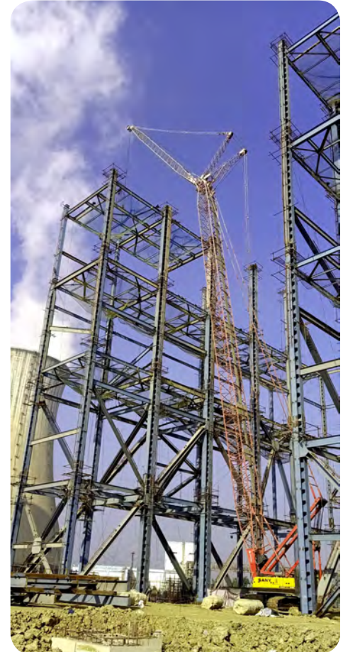
Sany SCC 2500 C (250 MT) crawler crane doing boiler structure erection at BHEL, Rajasthan
