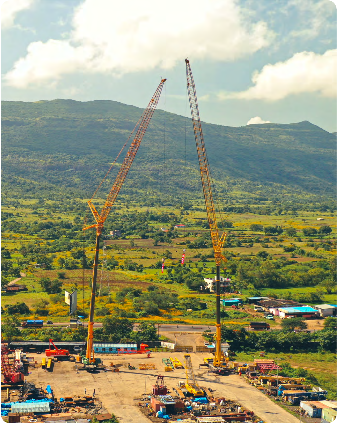
Aerial view of our Main workshop/overhauling Hub Vadgaon Maval, Sate, Pune
