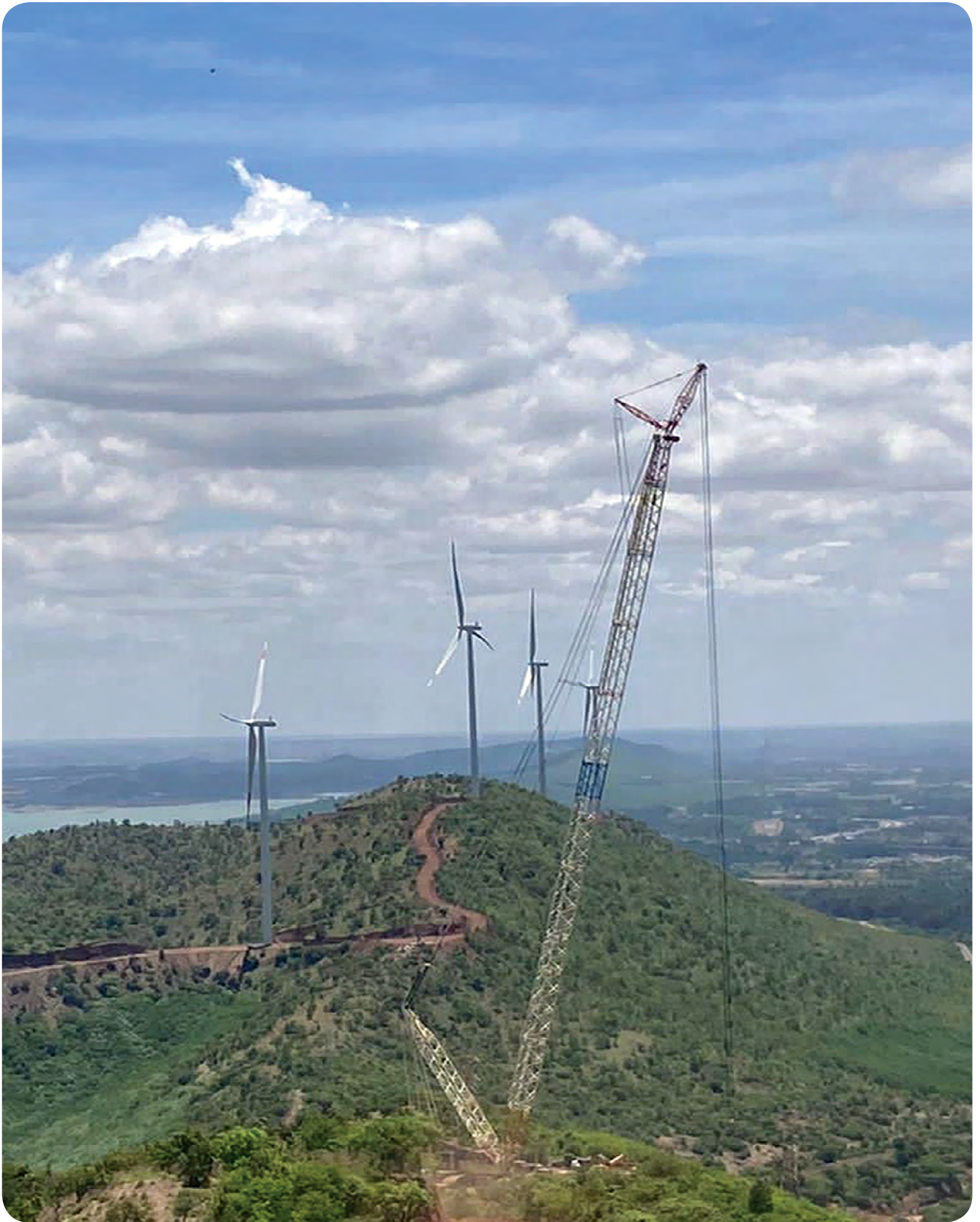
Terex CC2800-1 (600 MT Crane) in windmill configuration handling Nacelle 80 MT at the hub height of 120m Hospete, Karnataka
