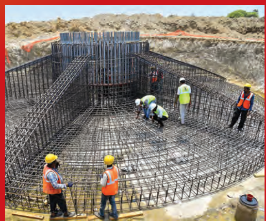
Wind Turbine Generator (WTG) Final Foundation at Sandur Karnataka
