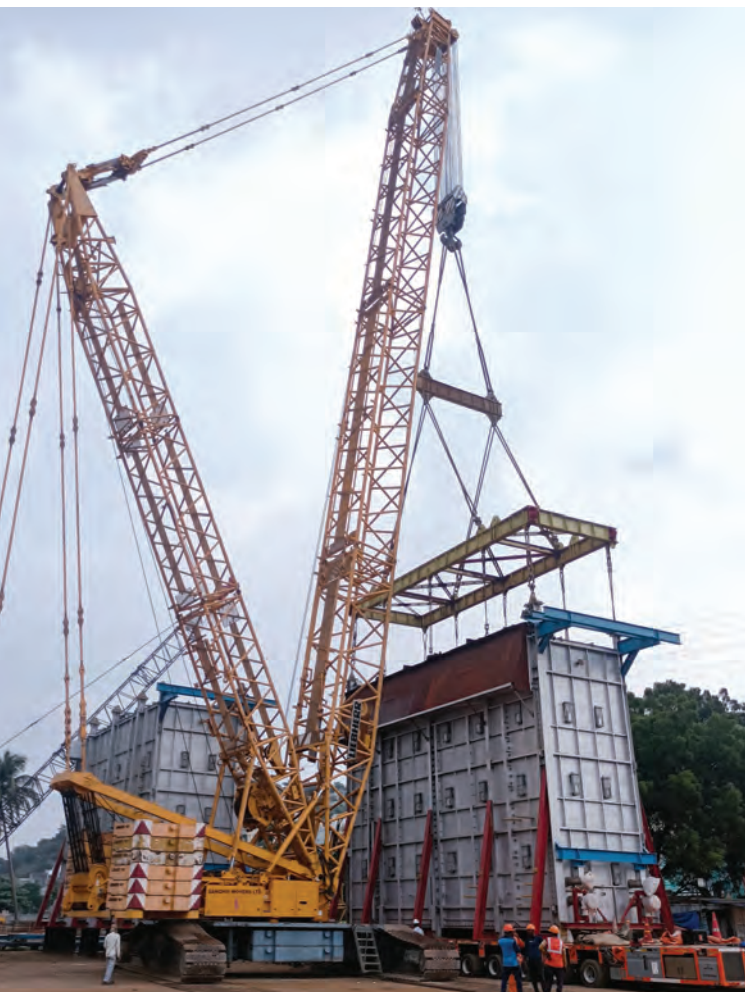
Liebherr LR 1400-2 doing heater module unloading job at HPCL Vizag
